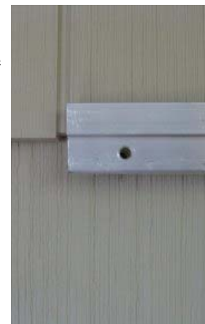
adjust to align holes w/ flat area
