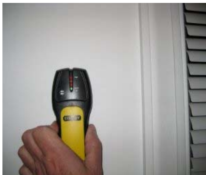
use a stud finder to locate studs from the inside
