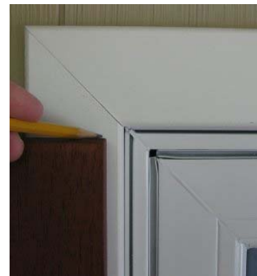
mark top of shutter on wall
