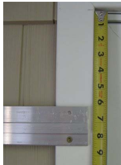
measure to top of mating brackets
