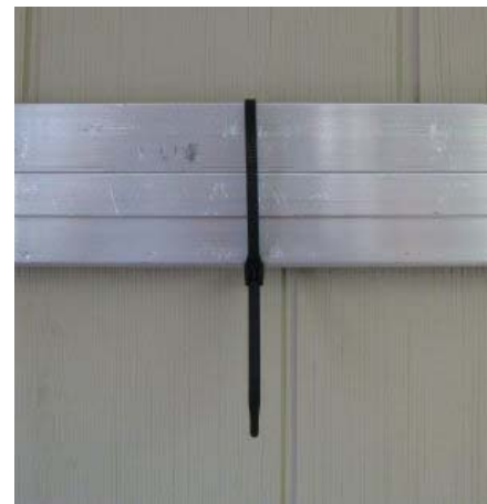
hang shutter and secure w/ cable tie
