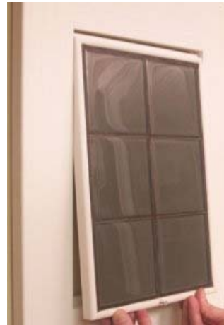
Step Three: insert new panel and tighten screw
