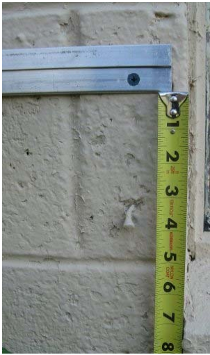
bottom bracket 7 inches up, then adjust to avoid mortar joints
