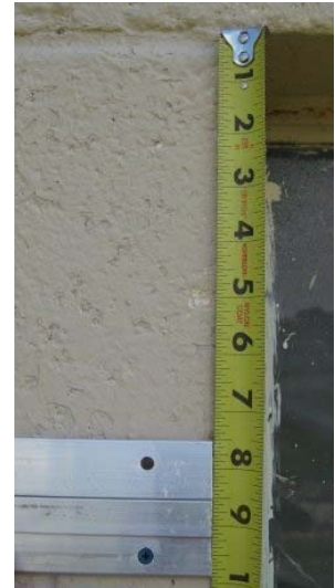
measure to top of mating brackets
