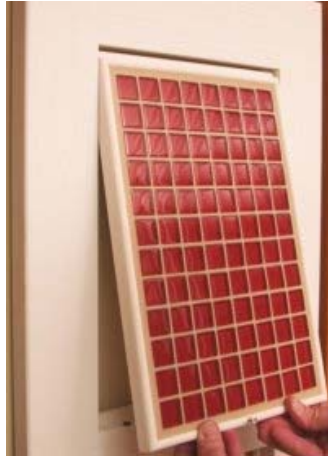
Step Two: lift panel out and down
