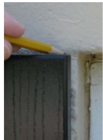
mark top of shutter on wall
