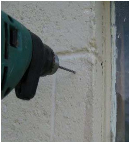
drill hole closest to window for Tapcon®
