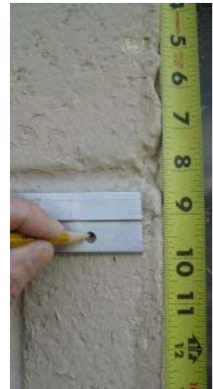
adjust to avoid mortar joints
